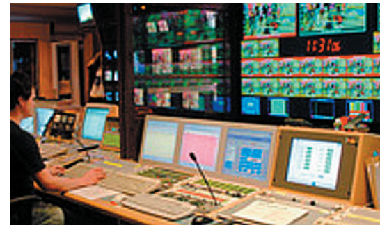
D-Series provides the most reliable and robust automation solution for any size multi-channel facility.
